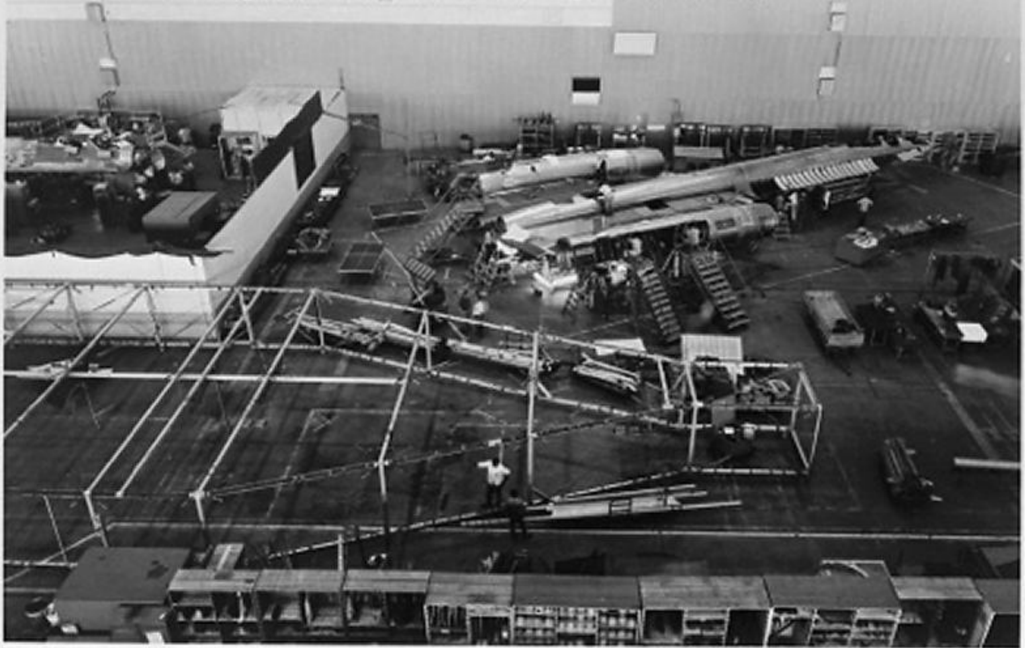
Carriage cover frame in work alongside A-12 Article #121
